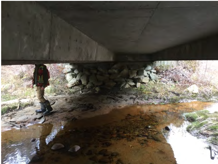
Right Bank Abutment when facing downstream
