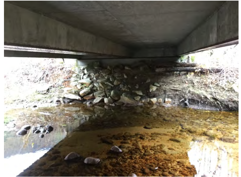
Left Bank Abutment when facing downstream
